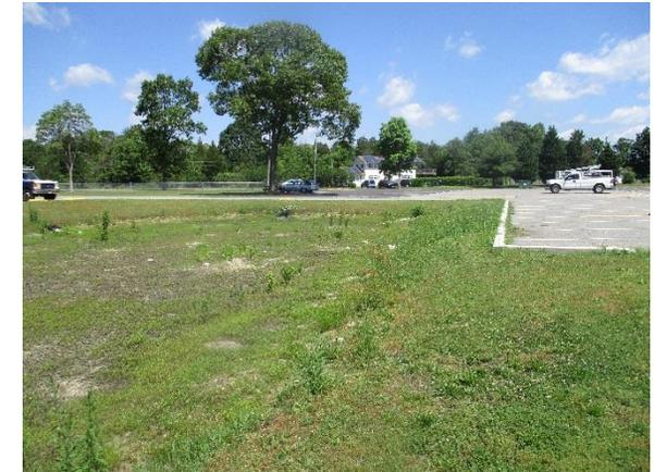
Stormwater is currently directed to an existing detention basin. Rain gardens adjacent to the building can capture, treat, and infiltrate roof runoff. A water harvesting system such as a cistern can collect rainfall from rooftops as well and be put to other use. A preliminary soil assessment suggests that the soils have suitable drainage characteristics for green infrastructure.
