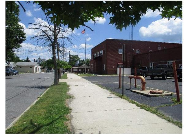
Parking spots west of the building can be replaced with porous asphalt to capture and infiltrate stormwater. A water harvesting system can be put in at the south end of the building to collect rainfall from the roof. A preliminary soil assessment suggests that the soils have suitable drainage characteristics for green infrastructure.
