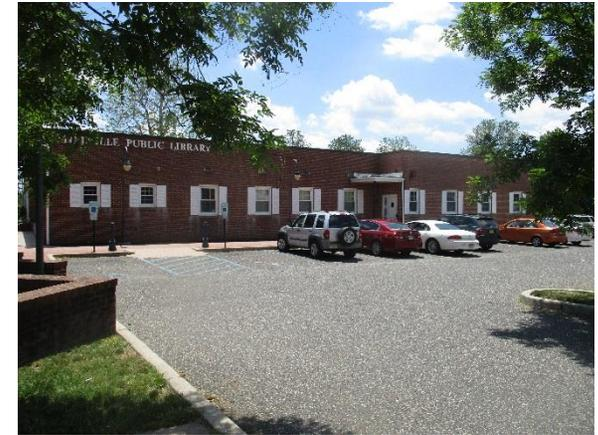
Parking spots north and west of the building can be replaced with porous asphalt to capture and infiltrate stormwater. A rain garden can be installed to capture, treat, and infiltrate runoff from the parking lot. A preliminary soil assessment suggests that the soils have suitable drainage characteristics for green infrastructure.
